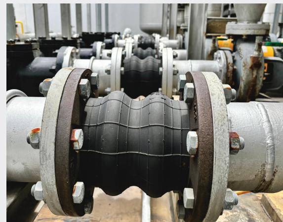
A flexible expansion joint connecting industrial pipes is engineered to absorb vibration and movement in fluid systems, enhancing stability and protecting equipment.
